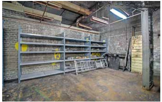
GPO equipment room. This is sadly the sum total of what was left when we cleared the room. The room is completely clear now, all the lino is up and it's ready for restoration.
